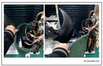
Fig. 109 Removing compressor cover 2
