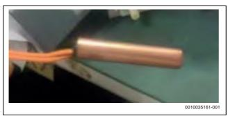
Fig. 132 Pipe thermistor
