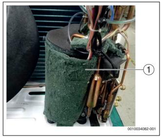
Fig. 108 Removing compressor cover 1
